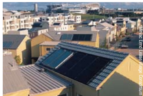
Newington village used a partially integrated PV system.
