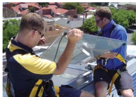
Installing semi transparent PV panels.
